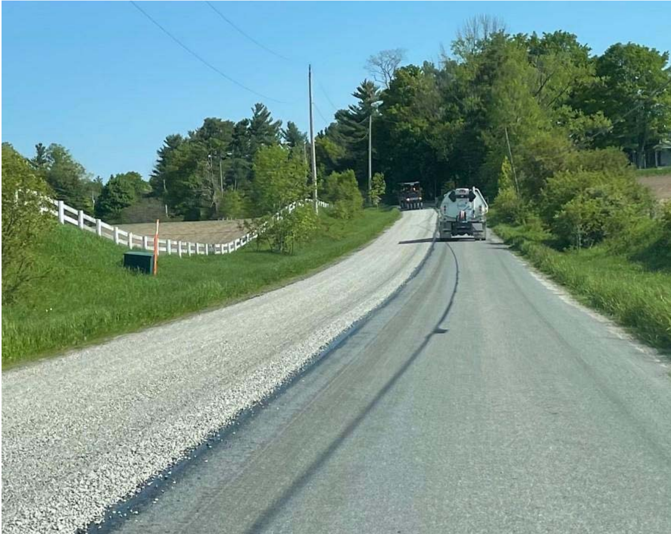
Image of a single surface treatment during construction
