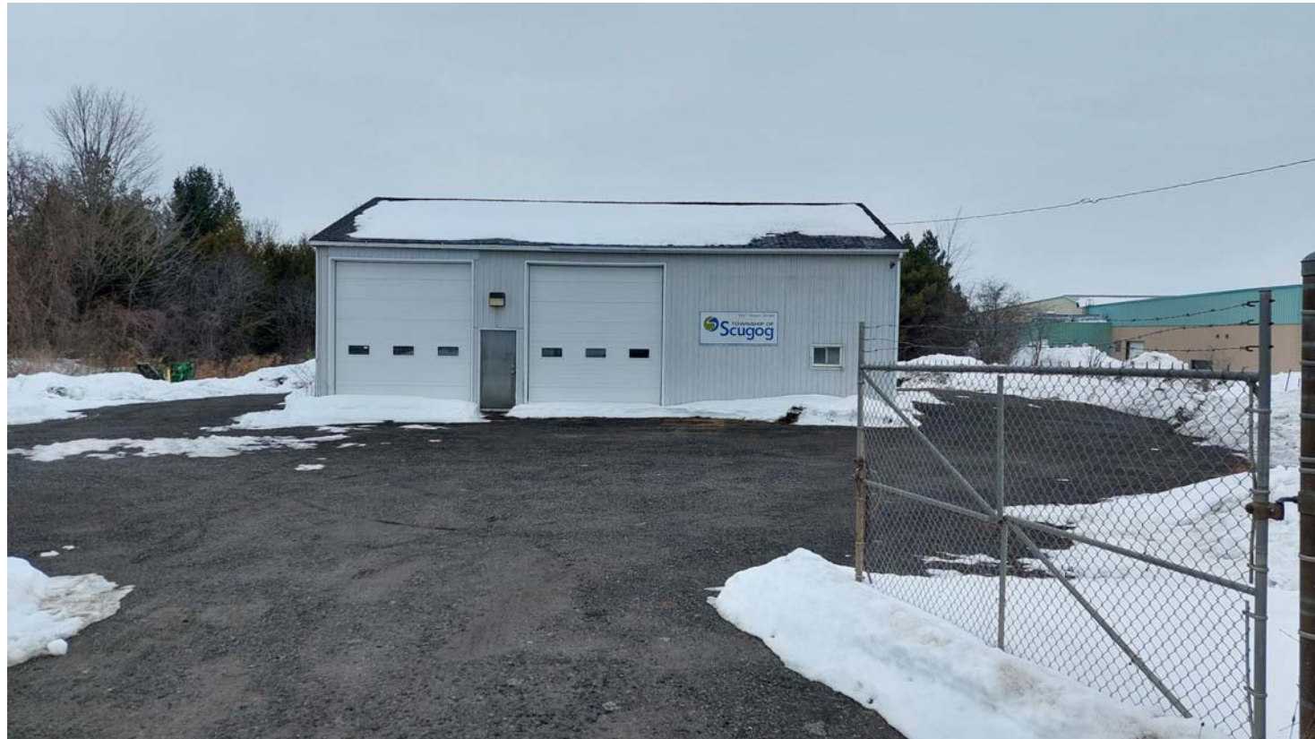
T:\Public Works and Infrastructure Services\Approved Projects\2024\Q2024-01 - Roof Replacement and Repairs 1647 Reach St\Photos\1000003052.jpg
